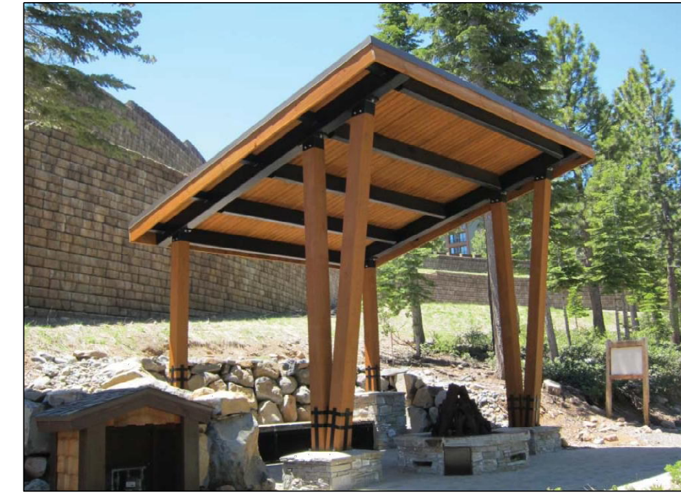
6 12' X 12' SHELTER LOCATED IN LINEAR & PICNIC PARKS, TYPICAL - SUBJECT TO CHANGE NOT TO SCALE
